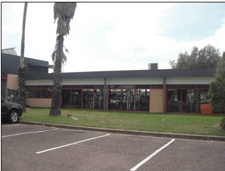
Figure 4: Existing gym building in southern area of the site
